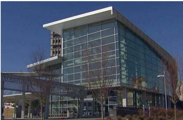
Durham Station Transportation Center. CTM provided painting inside and out and also furnishings.
